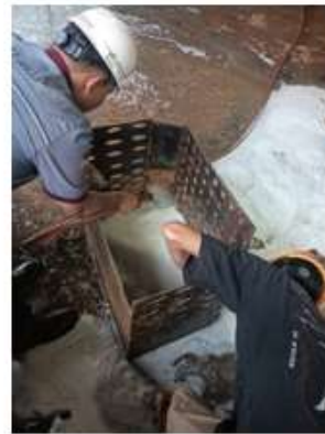
Figure 6. Installing the Pump Mount on the Strainer and Figure 7. Cleaning the Strainer
