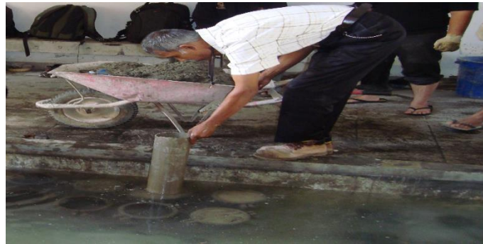
Figure 2.1 Method of casting in brackish water
