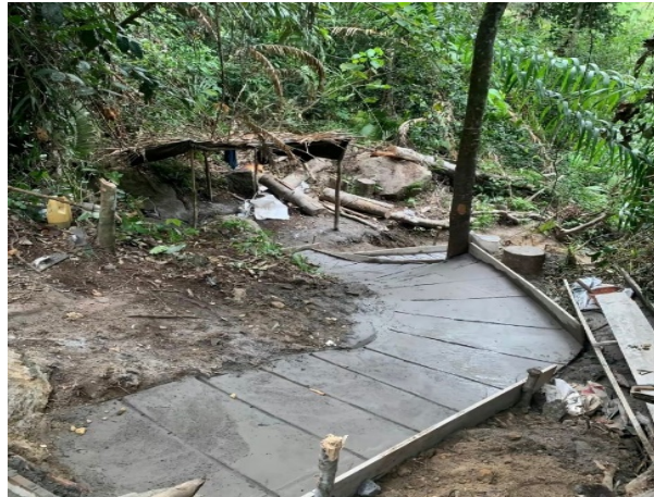
Figure 5. Road Access Repair
