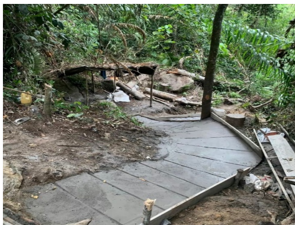
Figure 5. Road Access Repair
