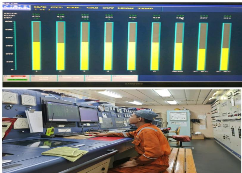
Figure 3.3 Turbocharger and Engine Control Room Indicators
