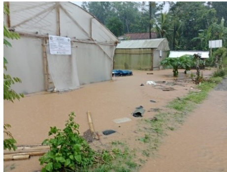
Figure 1. Condition of the greenhouse affected by the flood
